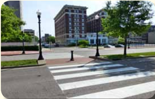
Figure 2.12: This high visibility crosswalk and median refuge island provides a safe connection across Riverside Drive to the Pigeon Creek Greenway and the Riverfront Esplanade.
