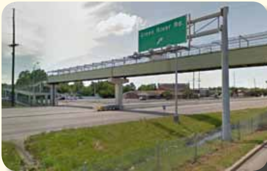
Figure 2.13: Overpasses, like this one at Cullen Ave over Lloyd Expressway, offer bicyclists and pedestrians safe crossing points over high-speed limited access arterials and increase route directness.
