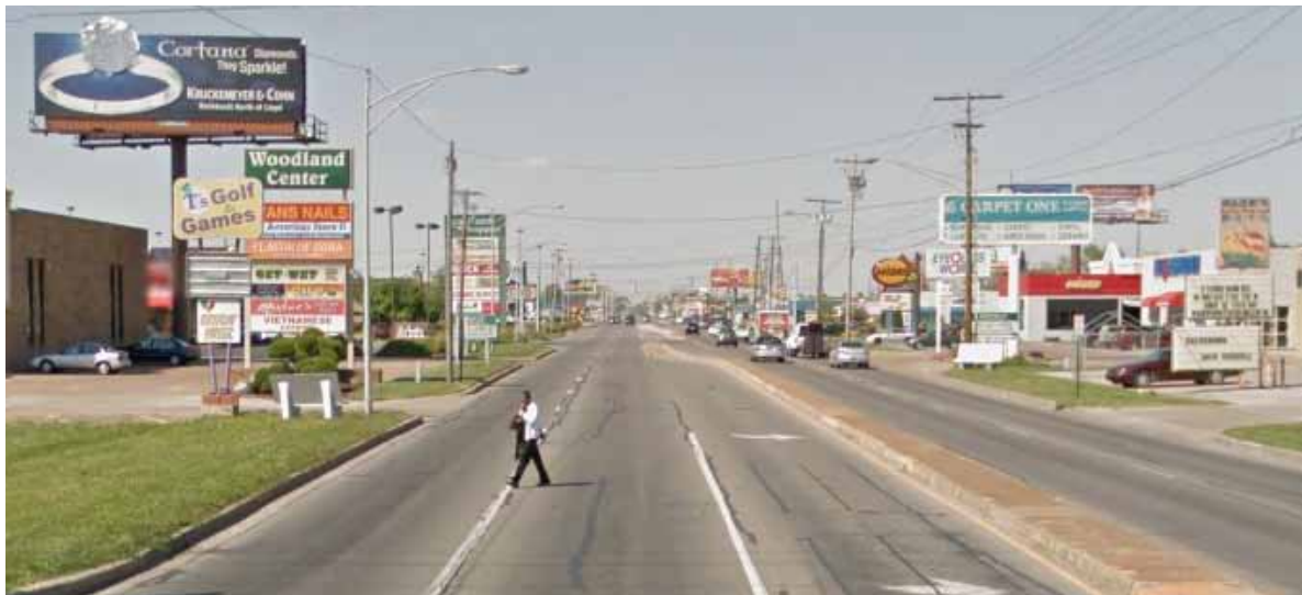
Figure 6.13: A lack of dedicated space for bicyclists and pedestrians creates unpredictable and unsafe behaviors.
