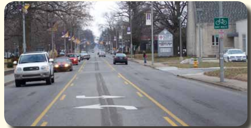
Figure 2.19: The road diet on Lincoln Avenue has helped to improve bicyclist and pedestrian safety and calm motor vehicle traffic.
